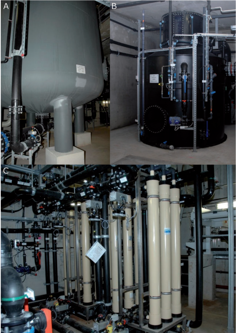
Figure 4: Typical life support systems of modern dolphinariums include drum filters (A), protein skimmers (B), and ultrafiltration systems (C). (Photos by Nuremberg Zoo)
